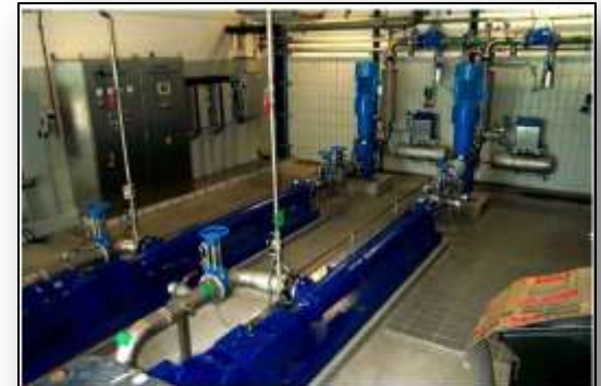
Crown Disintegrator Wiesbaden WWTP - 60m 3 /hr
