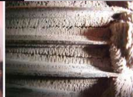
From SCS Energy
