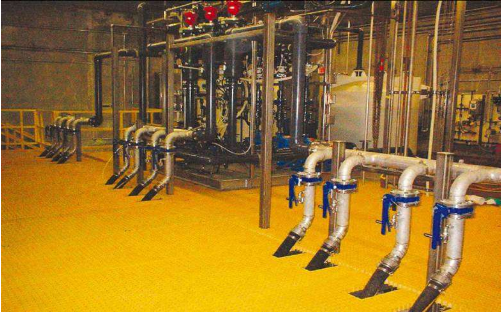
Concrete (In Ground) Membrane Tanks
