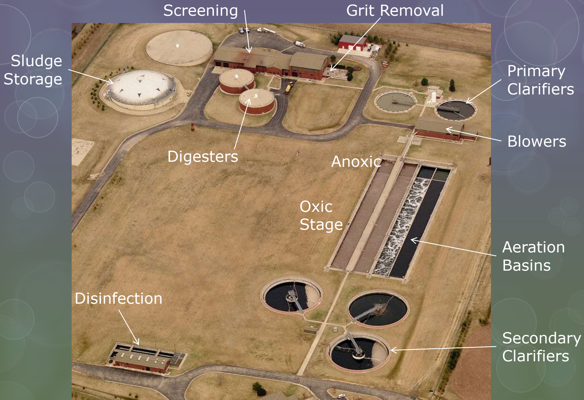
City of Beloit (WI) Water Pollution Control Facility
