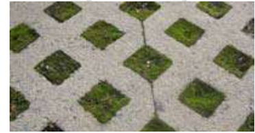
Concrete Grid Pavers (CGP)
