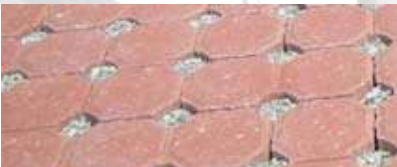
Permeable Interlocking Concrete Pavers (PICP)
