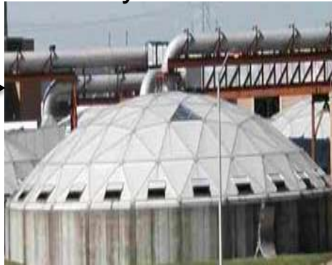
Gravity Thickeners
