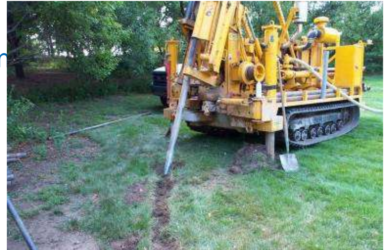
Track mounted CME-55 drill rig onsite
